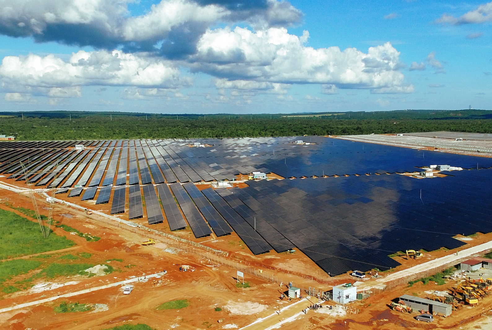
An aerial view of the Bangweulu Solar Photovoltaic power plant in partnership with NEOEN/First Solar in the Lusaka South Multi-Facility Economic Zone. 📷 IDC
