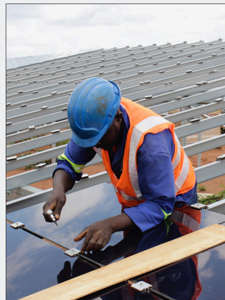
A technician installs solar panels at the Bangweulu solar park during construction phase.
