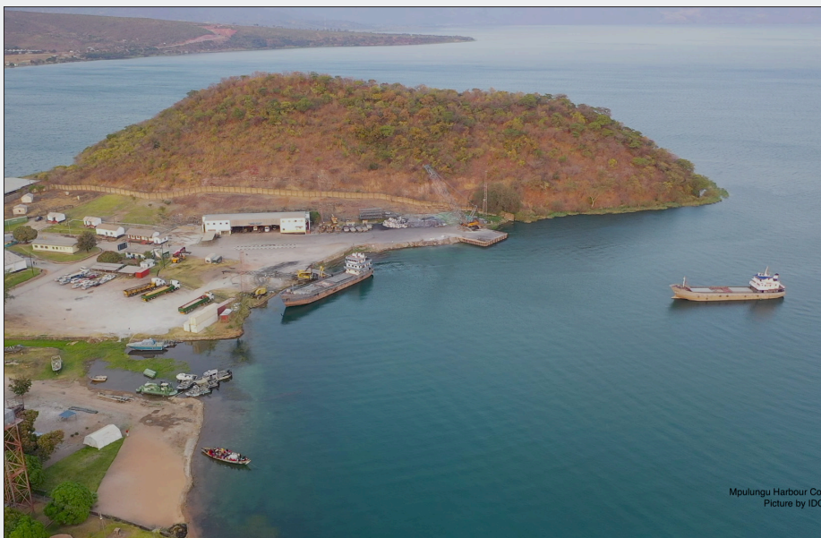
An areial view of Mpulungu Harbour Corporation Limited. The company recorded a profit for the first time in 2017 as a result of the IDC's transformation programme.
