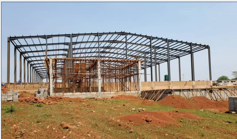
The IDC is constructing a fruit processing plant in Katete District. Due for commissioning in 2021 Q1, the project will provide a ready market for mangoes and citrus fruits that usually go to waste in Katete and surrounding districts.
